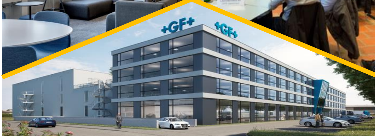
New facility Biel
